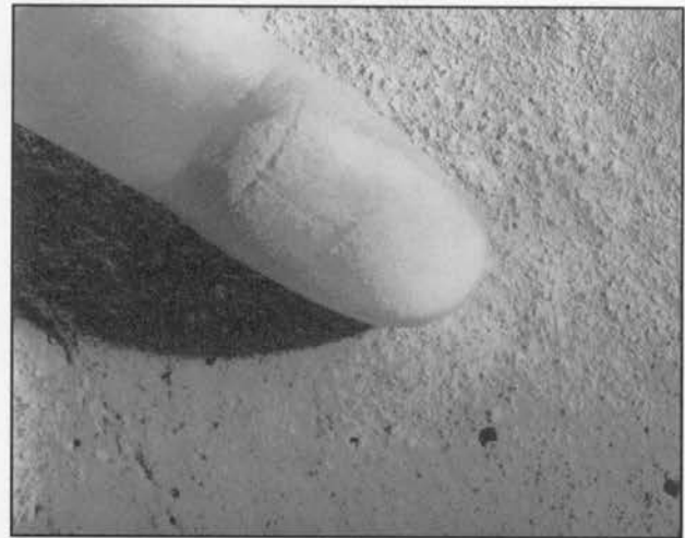
Dusting concrete surface
