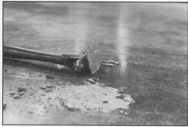
Delaminated Concrete
