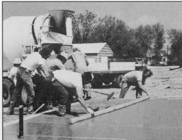
Finishing Concrete Flatwork
